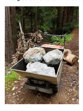
A rock wall was built in the narrow spots and on the switchback turn with the trail building machine. Notice the opposable thumb on the grip.
