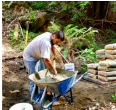
All the concrete for the foundations had to be hand-mixed, see large stack to right, they earned their money that day!
